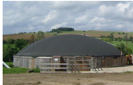
Figure 10. Photo APESA, installation du GAEC Oudet
